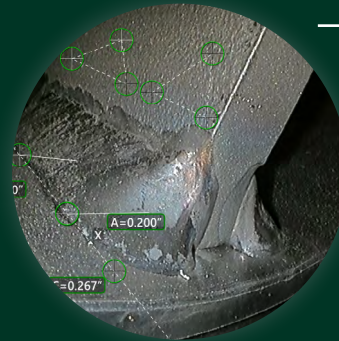
Weld (General Inspection)
